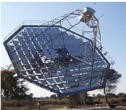
Fig 7. Arun dish based solar cooker (By IIT Bombay 2014)
