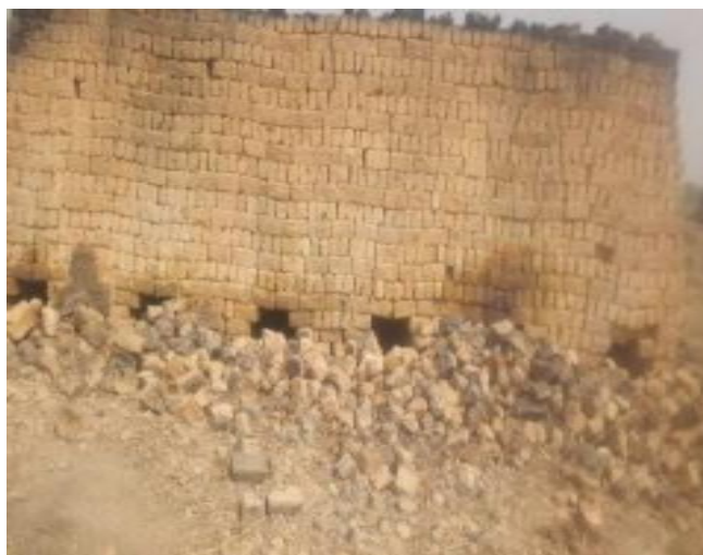
Fig 2: already burnt bricks
