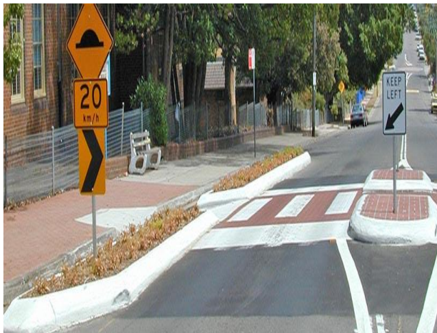
Figure 11. Kerb extension (Source: http://www.roadsafety/wp-content/uploads/2016/07/pedrefugeilsand.jpg )
