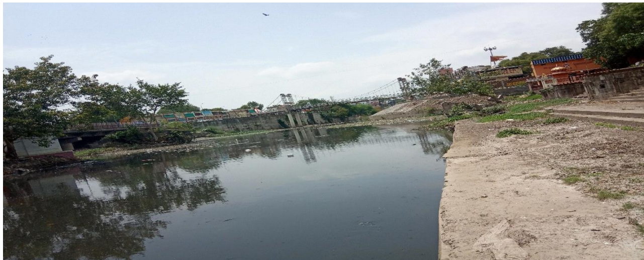
Figure: 2: View of Khan River in Indore city at Krishanpura Bridge
