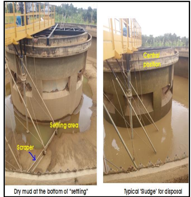
Figure 11: Drained Clarifier Depicting Settled Mud
