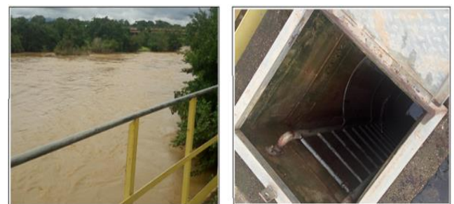
Fig. 1: Mada River (left) and Intake Structure (right)
