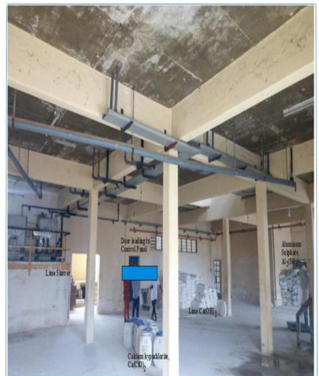
Figure 5: Chemical Building showing the Chemical Store
