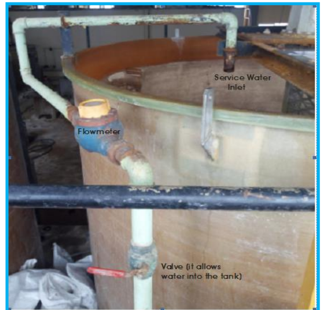
Figure 6: Service water inlet to Alum Tank
