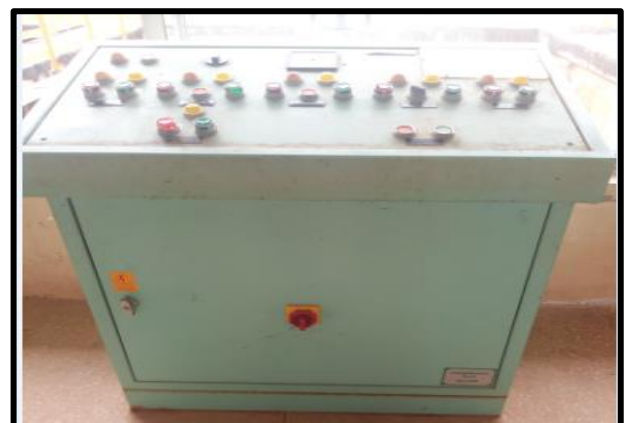
Figure 23: Filter Control
