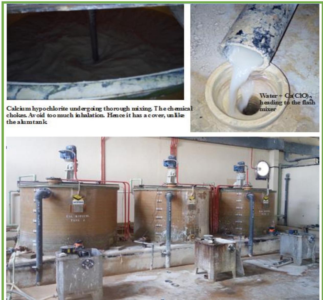
Figure 14: Chlorine Tanks
