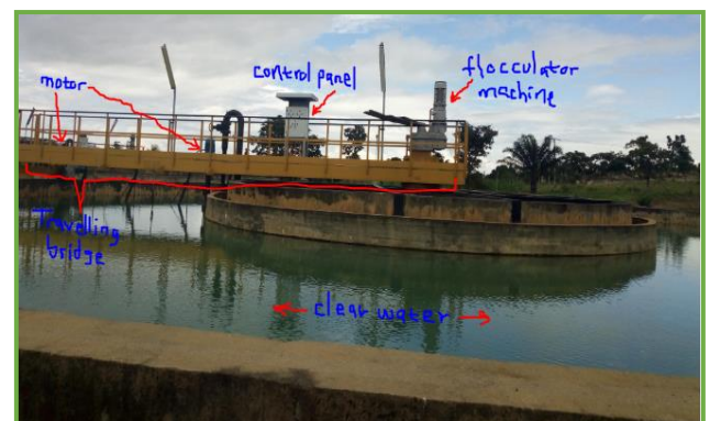
Fig. 16: Features of the Clarifier
